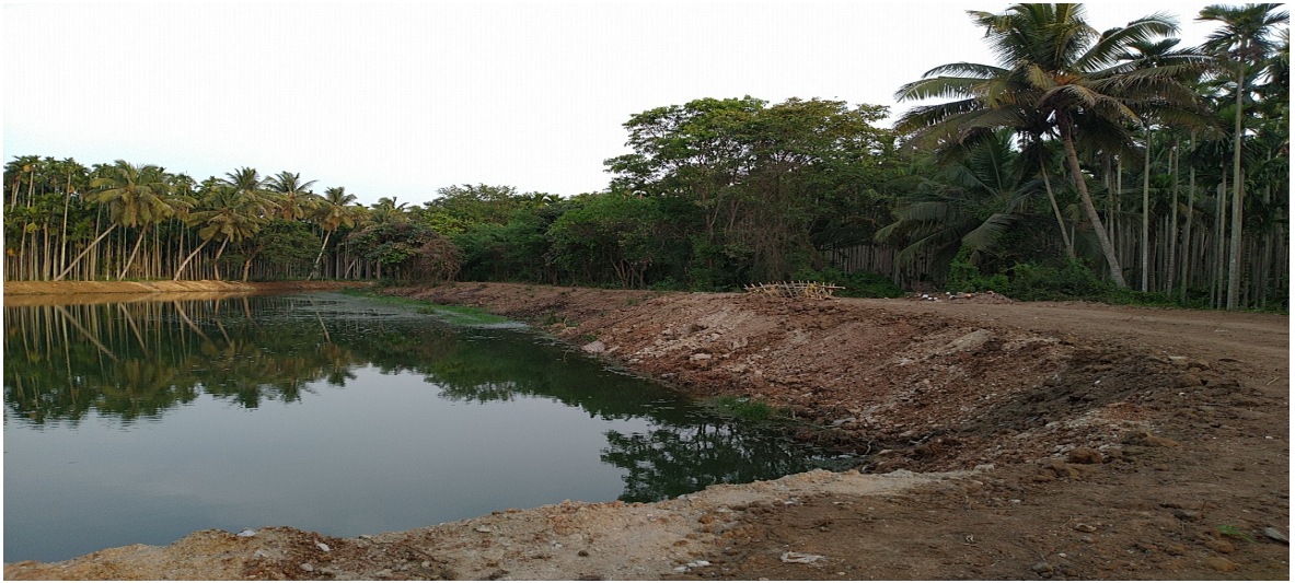
23-05-2019 Our volunteers cleaned and joined their hands in renovating the ancient water tank for “Rain Water Harvesting” at Yalavatti village in Shivamogga taluk. Programme Officer headed the team of volunteers.
